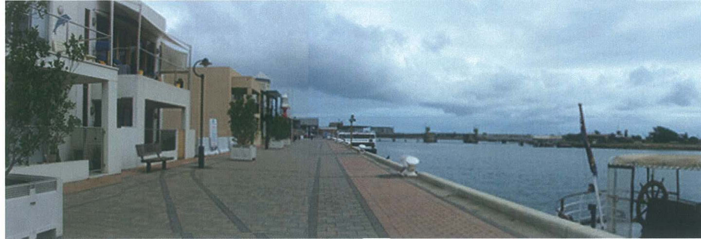
View looking west down McLaren Wharf
