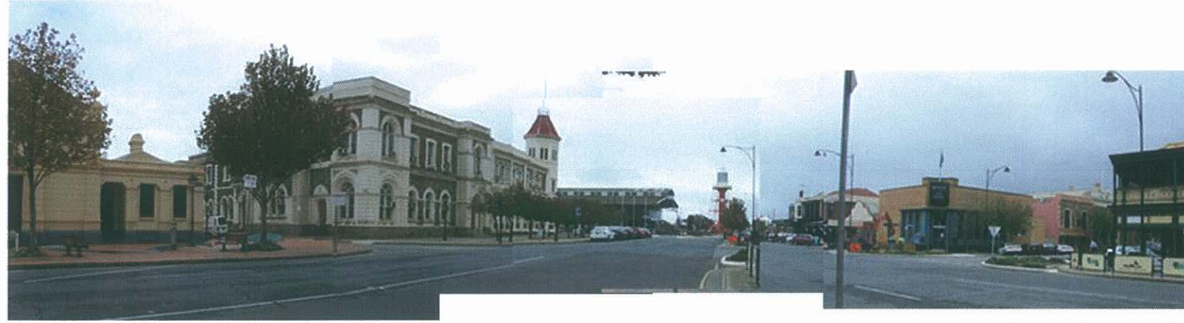
View of Customs House, Lighthouse and Black Diamond Square looking north down Commercial Road
