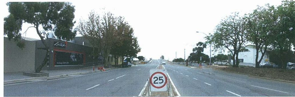
View of Birkenhead Bridge looking north.
