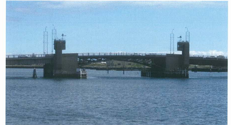
Figure 4 Birkenhead Bridge (in its present form) linking McLaren Wharf and Cruickshank's Corner Precincts
