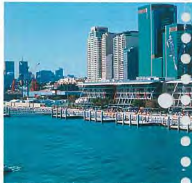
King Street Wharf Redevelopment Sydney NSW
