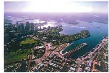
Finger Wharf Redevelopment Woolloomoo NSW
